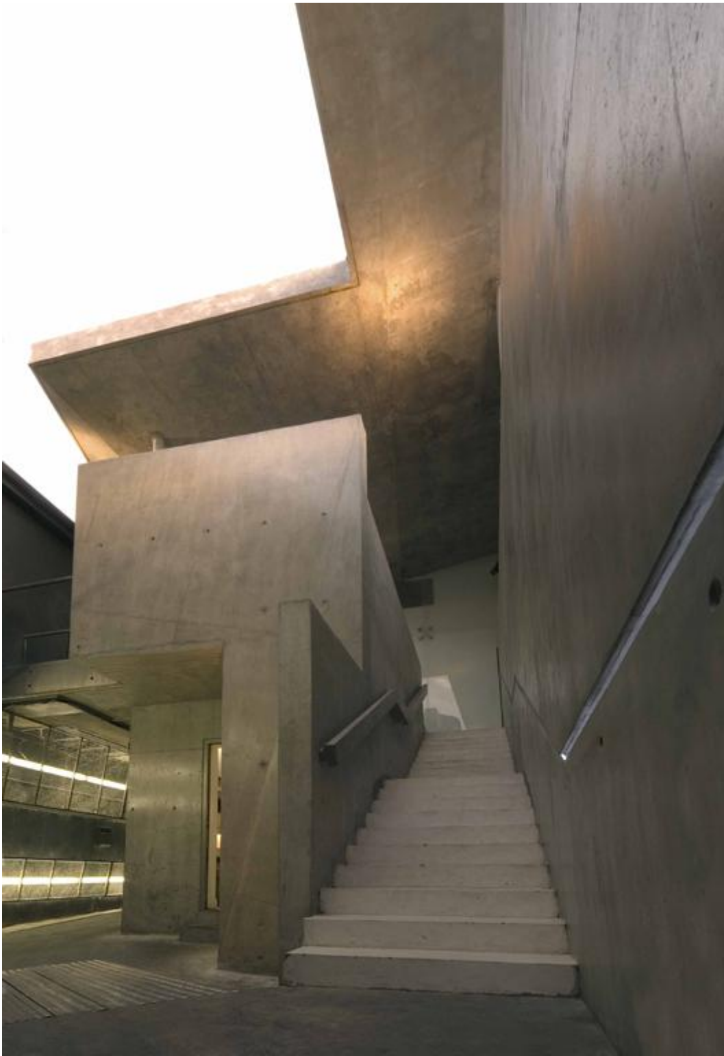
Solid Cast Concrete Stair rising to External Terrace with Oversailing Folded Canopy
